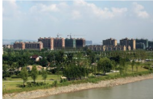
Commercial and residential development underway on the Sino-Singapore Nanjing Eco Hi-tech Island
